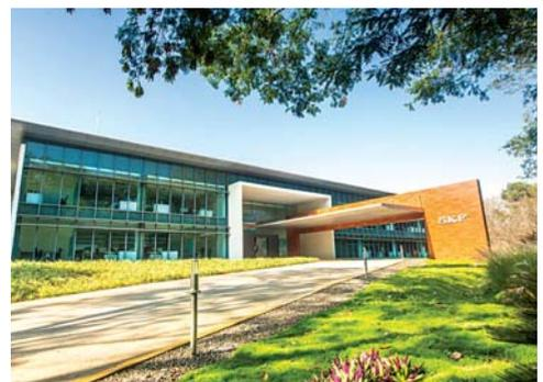
Designed with a focus on energy and water efficiency, the building's envelope material and lighting help it exceed LEED's baseline building standards by approximately 60 percent. In total, 65 percent of the building's electricity comes from roof-top solar panels and at peak office hours, it is energy neutral, as 100 percent of its power requirement is drawn from solar energy. Sh-
