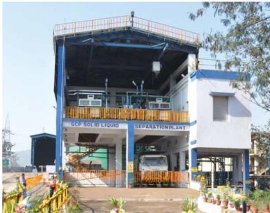
the processing of GCP slurry will be fully recycled, leading to water conservation to the tune of 15 cubic metre per hour.
